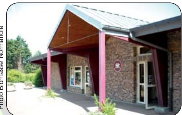
Photo Biomasse Normandie
